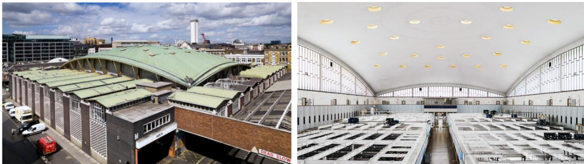
Figure 1 – Smithfield poultry market exterior (left) and interior (right) © Historic England Archive
