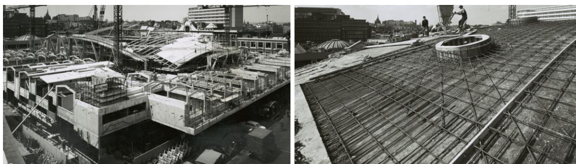
Figure 4 – Construction of the market roof in the 1960s © John Maltby
