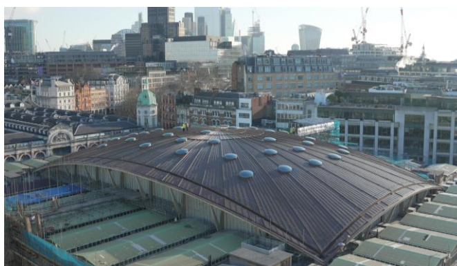
Figure 11 - New copper finishes on the roof (taken March 2024) © FMJ Limited
