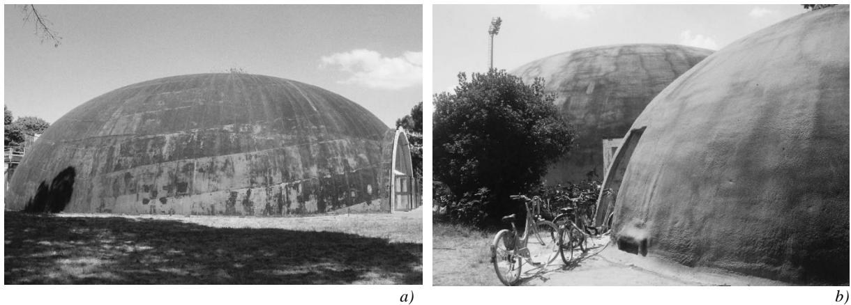
Figure 8: a) Indoor swimming pool designed with the Binishell construction method in Prato (1977); b) 'Le Cupole' sports facility, Castelfranco Emilia (Modena) (1977); pictures from Mellone [4].
