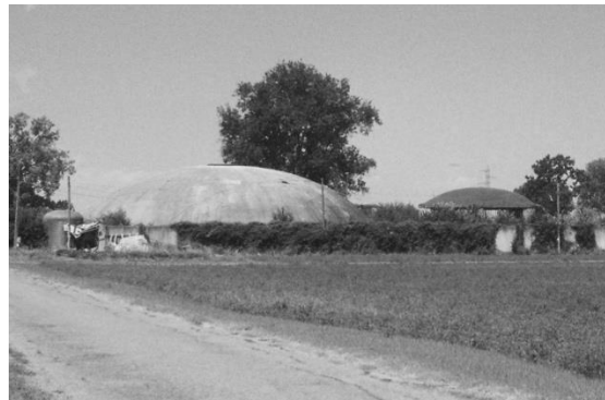
Figure 2: D. Bini, the Binishell experimental field in San Cesario sul Panaro (Bologna), Mellone [6]
