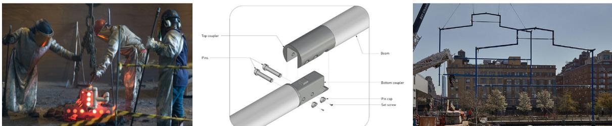
Figure 12 – Casting of the “nodes,” diagram showing the “coupler” connection, erection of the steel frames
