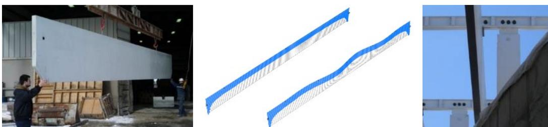
Figure 7: Corning Museum of Glass Art and Design Wing: at Béton Préfabriqué du Lac (left); analysis model (center) and “stanchions” on top of hollow concrete walls (right).
