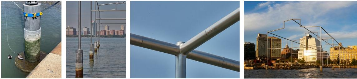
Figure 11 – Corrugated concrete column base with algae, column base connection, column node and column-to-beam “coupler” connection, and completed structure as seen from the river
