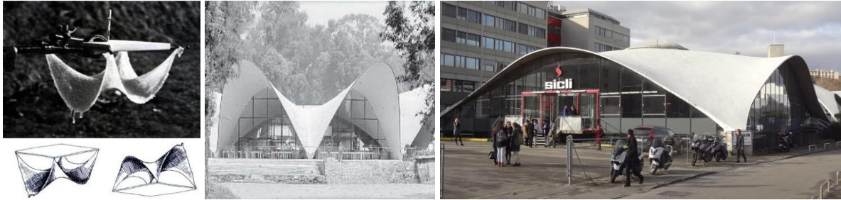
Figure 4: Heinz Isler's Frozen Sheets, Félix Candela's Los Manantiales Restaurant in Mexico (1958), and Heinz Isler's Sicli Pavilion in Geneva (1969) [[3], MHM55]
