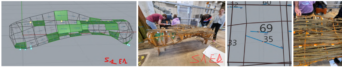
Figure 25: For La Vague : (a) one step of braiding needs during the filter operation, (b) braided shell after this step, (c) zoom on braiding plan, (d) wicker mesh in orange and cells number marks.
