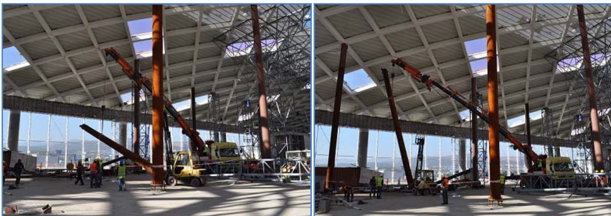
Figure 7: De-propping of typical circular prop
