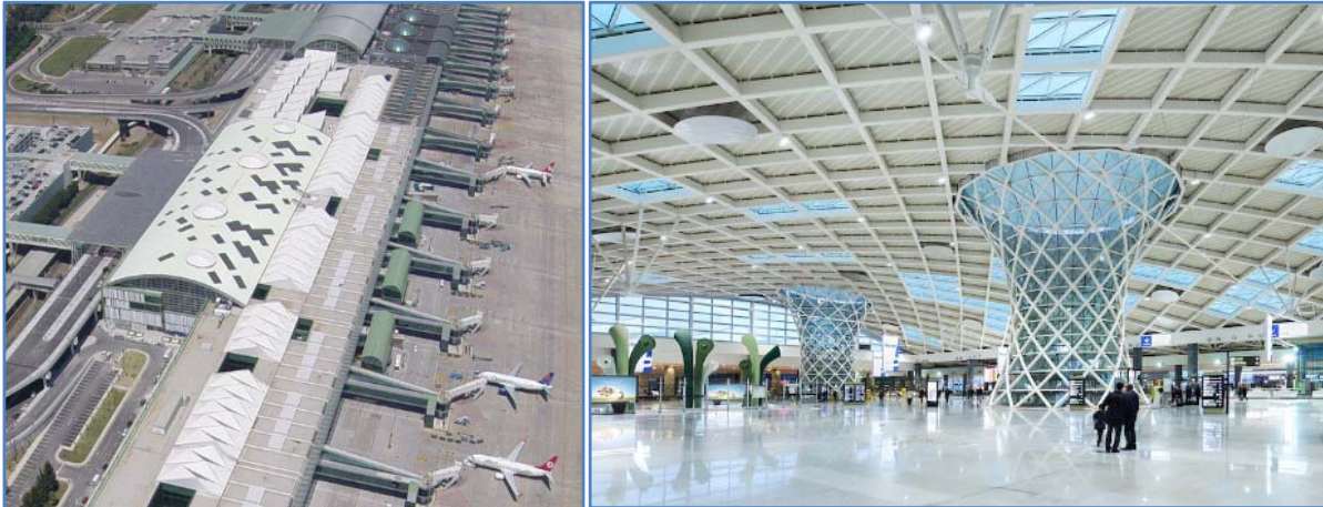
Figure 14: General outside and inside views from the completed project
