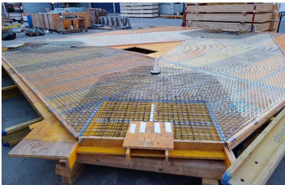
Figure 3: Formwork and reinforcement
