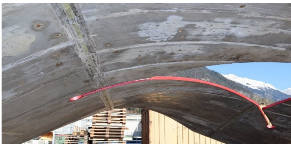
Figure 7: Actively bent concrete shell – bottom view
